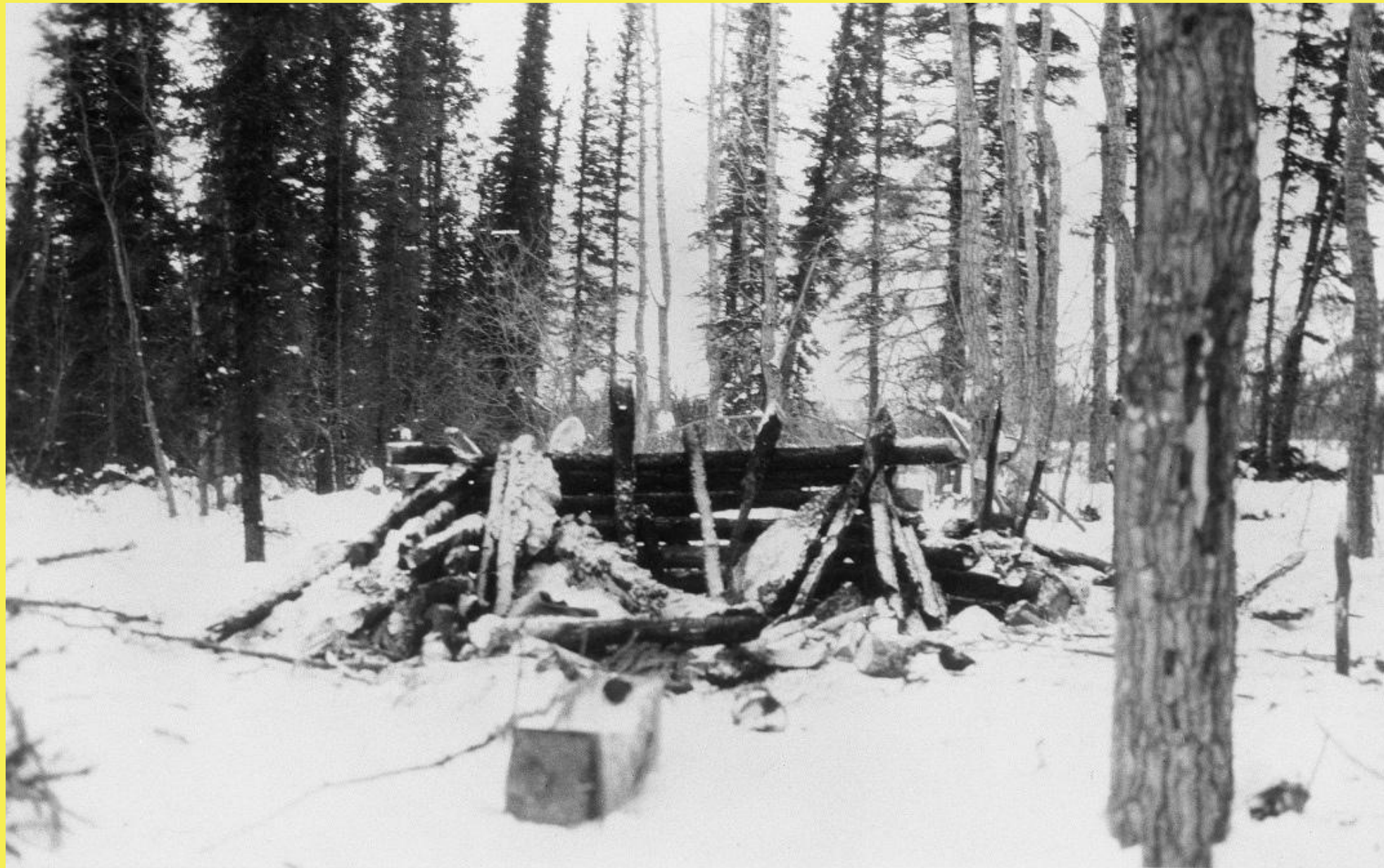
JOHNSON'S CABIN AFTER IT WAS DESTROYED
